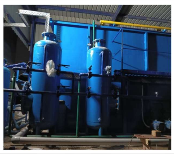
50 KLD E.T.P PLANT VANDE BHARAHT TRAIN,DEPOT DELHI. INDIAN RAILWAY
