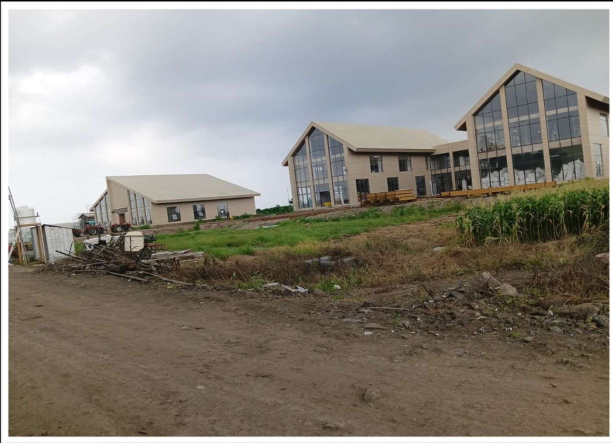
50 KLD WATER TRETMENT PLANT TAFE J FARM BHAWANI MANDI KOTA RAJASTHAN
