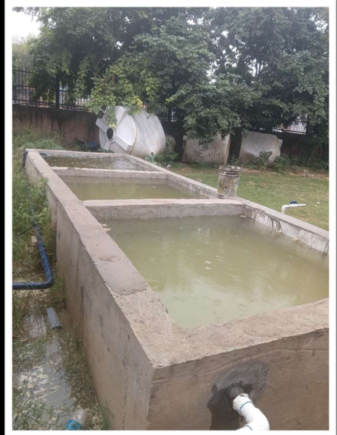
150 KLD S.T.P PLANT RAJ BHADUR MEMORIAL GOVT. HOSPITAL BHARTPUR RAJASTHAN
