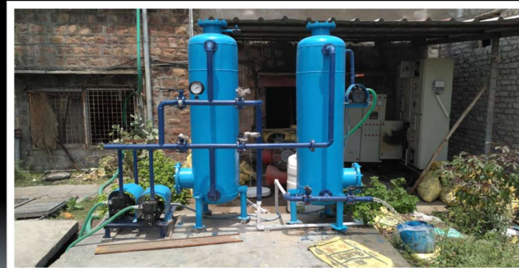
W.T.P RAILWAY LAUNDRY, KOTA, RAJASTHAN
