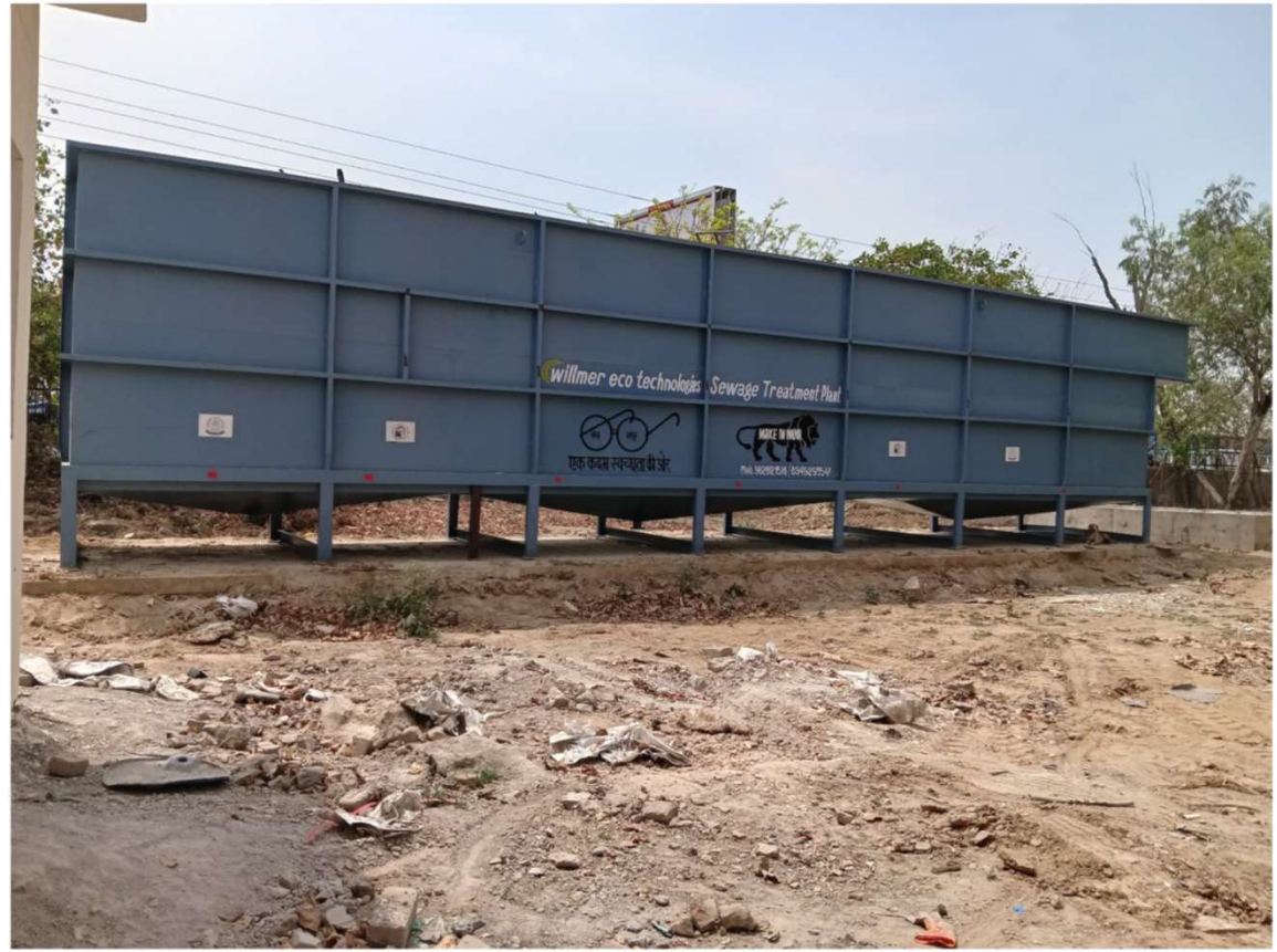
150 KLD S.T.P PLANT RAJ BHADUR MEMORIAL GOVT. HOSPITAL BHARTPUR RAJASTHAN
